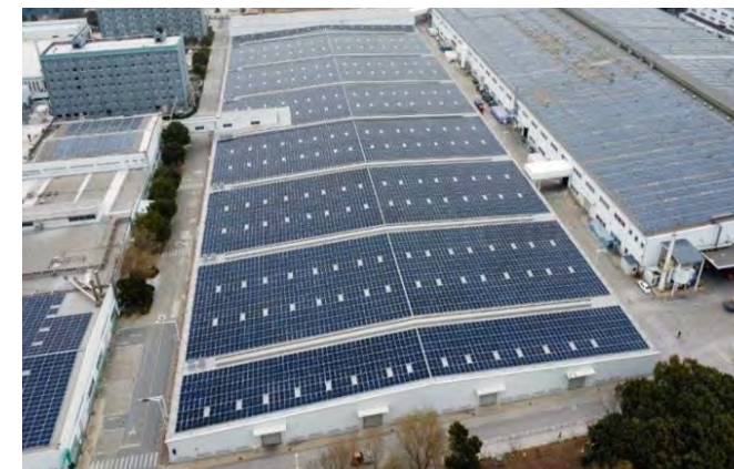
Rooftop Photovoltaics at the Hisense Huzhou Air Conditioner Factory
